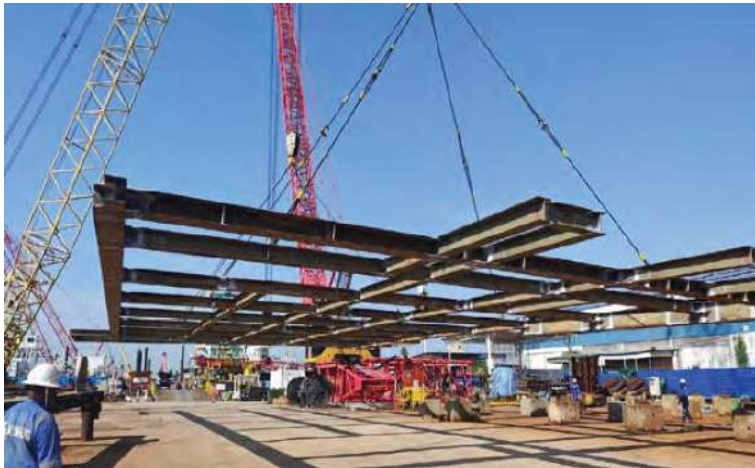
FPSO Module Fabrication at Kim Heng Yard
