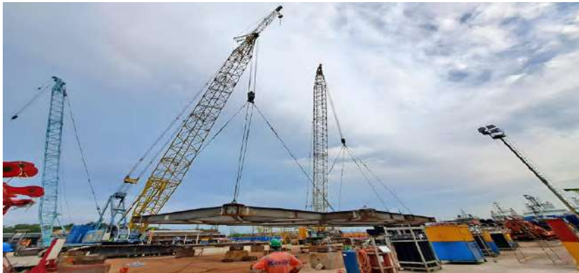
Fabrication of Steel Modules: Dyna-Mac Collaboration
