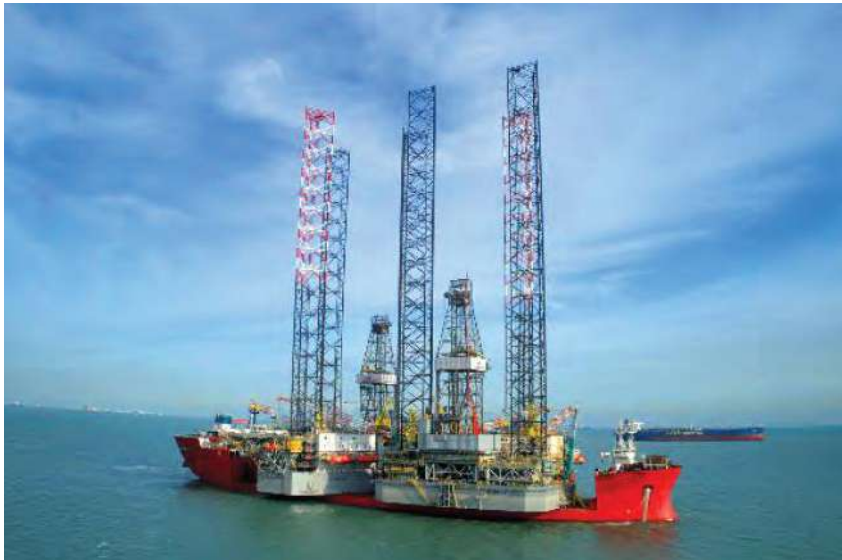
Rig Reactivation Works
